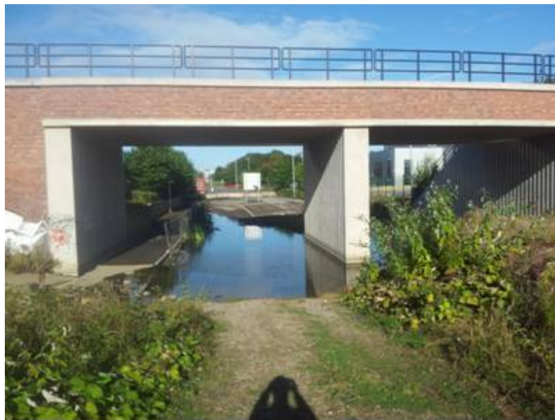
Photo 5 – Looking Westbound towards A461 (Walsall – Stourbridge line bridge shown)
