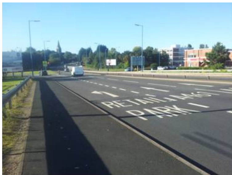
Photo 1 – Left Turn Filter (A461) – looking southbound from M6 Junction 9
